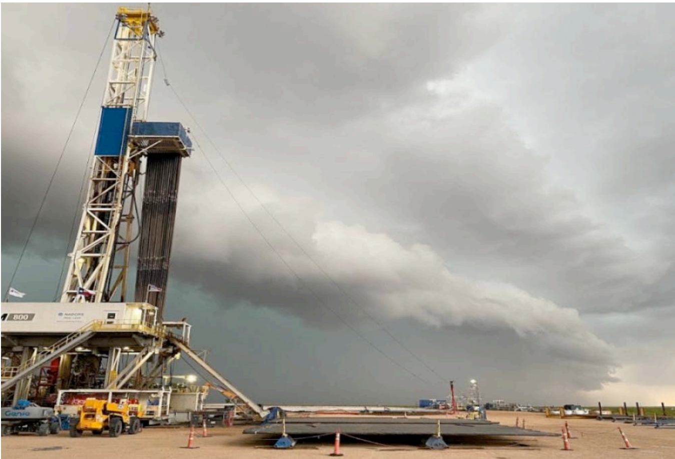
Drilling in the Permian Basin has been an area of focus for U.S. Energy Development Corp. Pictured is the Nabors 1206 Storm rig. (Source: U.S. Energy Development Corp.)
